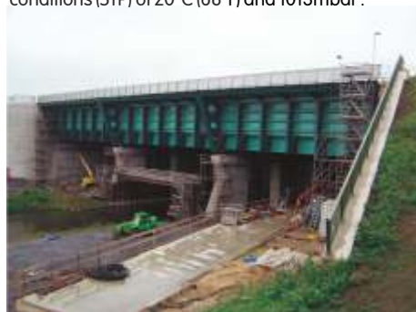
channel bridge Lippe 2006
