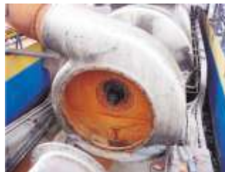
coating of a pump housing
