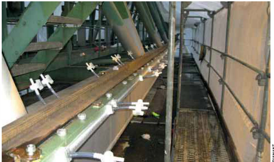
Filling the gap with the liquid shim and final assembly of the crane rail.
