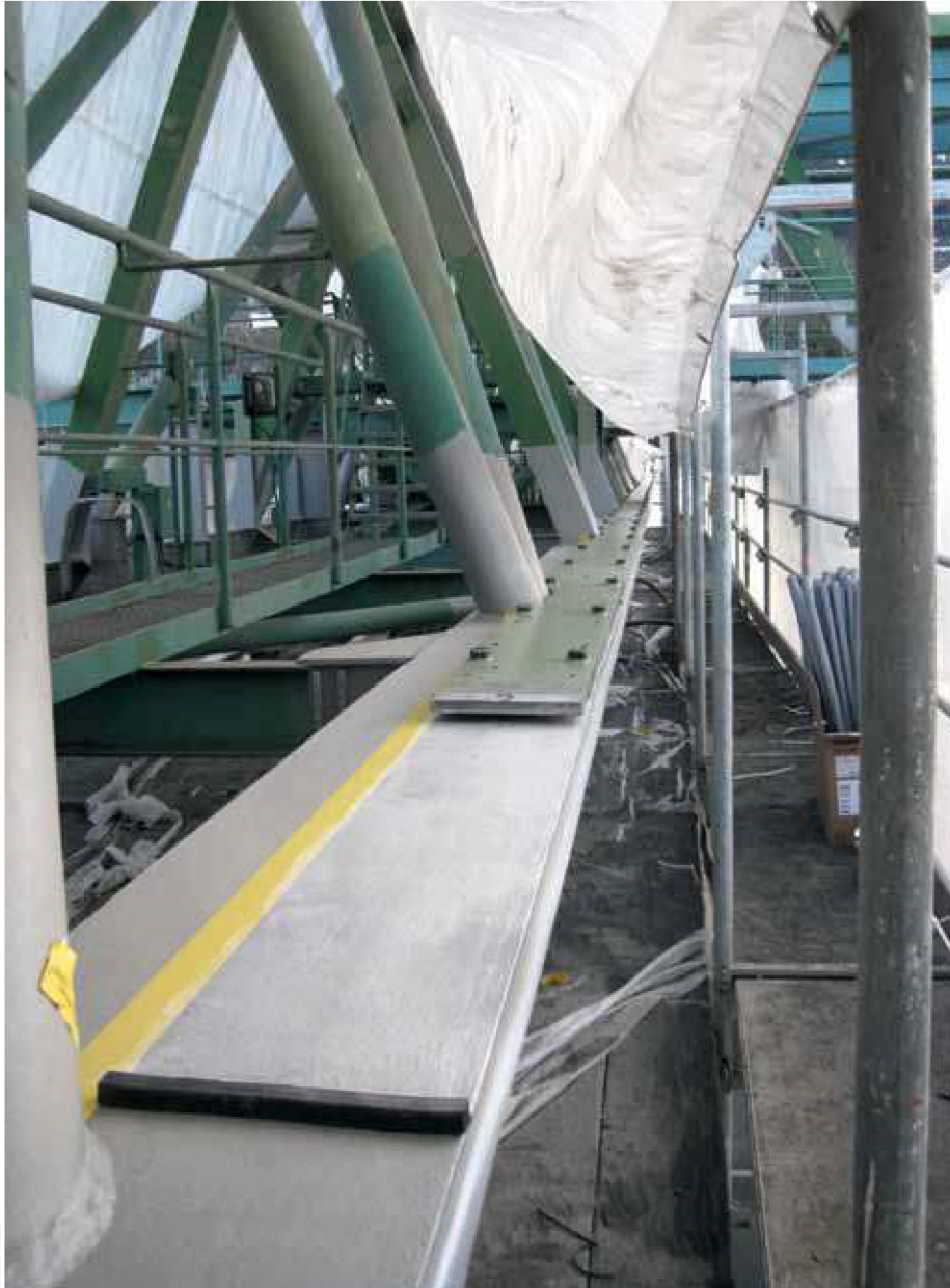
Attaching the new rail support with a visible gap to the existing support.
