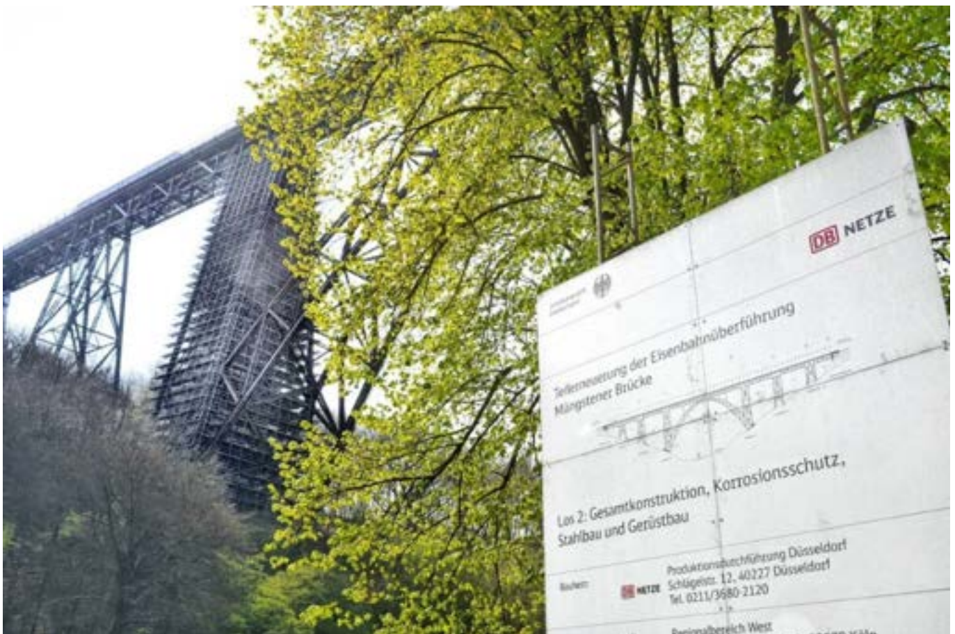
Figure 3: The refurbishment work began in 2013
